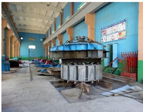
Photo 16. Out-of-service pump units of GPS-1 (left) and GPS-2 (right)
