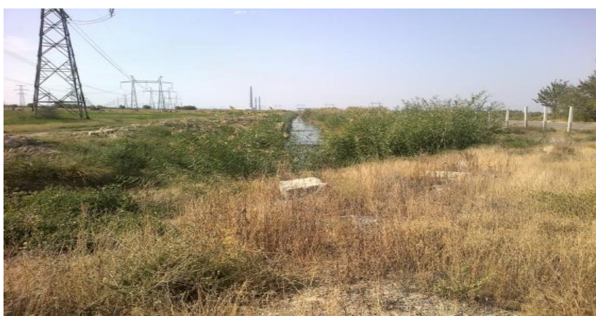
Photo 12. Condition of the Zafarabad DNW
