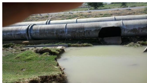
Photo. 18. Failure on the TM-2 canal (left) and blowout in the GPS-1 pressure pipeline.
