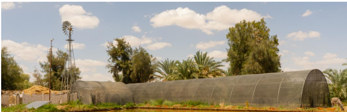
Figure 2: Picture of the shade house model installed in El Heiz oasis with solar panels showing on the left, the shorter section of the L-shaped greenhouse housing the fishpond, the crop production housed in the longer part of the shade house.
