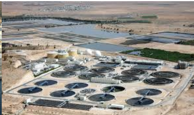
Kherbet El-Samra WWTP - Jordan
