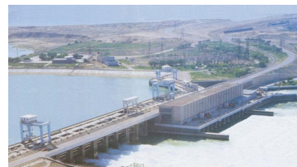
Tuyamuyun Hydroelectric Complex, Ilkhom Zhuraev
